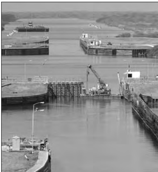
TOUGH TRIP: Workers on a barge use scaffolding to access and repair the lock gates in Matagorda. Access to West Matagorda Bay is restricted, and anglers are asked to call the lockmaster before planning their trip. Photo by Mike Price for Lone Star Outdoor News.
