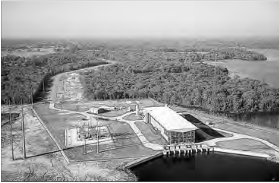
PUMPED UP: A new water pump station at Lake Fork cost the city of Dallas more than $200 million, including the pipeline connecting the station. Photo by the city of Dallas.
